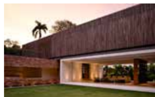
3A King Albert Park Singapore Residential Architecture
