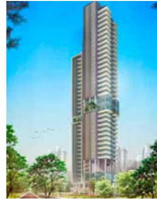
Residence 28 Condo Jakarta, Indonesia Residential Architecture, Interior Design, Landscape
