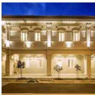
Koon Seng Road Shophouse Singapore Residential Architecture
