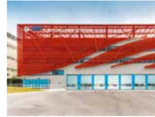
Jurong Fire Station Singapore Civic
