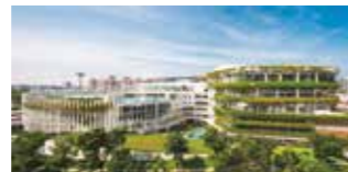
Heartbeat@Bedok Architecture, Landscape, Lighting and M&E Engineering BCA Universal Design Mark Awards, GoldPlus
