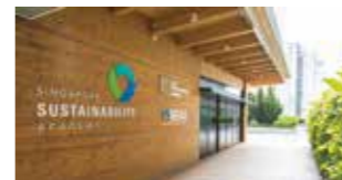
Singapore Sustainability Academy Architecture and M&E Engineering BCA Green Mark Awards, Platinum
