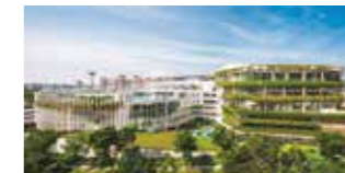
Heartbeat@Bedok Architecture, Landscape, Lighting and M&E Engineering SILA, Silver
