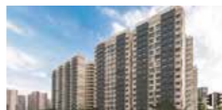
West Rock @ Bukit Batok Architecture, Landscape, C&S Engineering and M&E Engineering BCA Universal Design Mark Awards, GoldPlus
