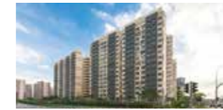
West Rock @ Bukit Batok Architecture, Landscape, C&S Engineering and M&E Engineering SILA, Silver
