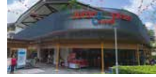
Jurong Central Plaza Architecture, C&S Engineering and M&E Engineering HDB Design Awards, Rejuvenation category, Certificate of Merit
