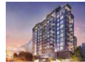
Haus on Handy M&E Engineering BCA Green Mark, GoldPlus
