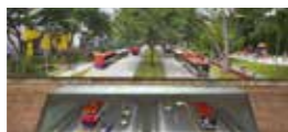
North-South Corridor (Tunnel) Between Ang Mo Kio Ave 3 and Ang Mo Kio Ave 9 Architecture BCA IDD Awards, Project Category, GoldPlus
