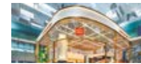
Changi Airport Terminal 3 Central, Lotte Duty Free Project Management Asia Pacific Property Awards, Commercial Redevelopment/Renovation, Singapore
