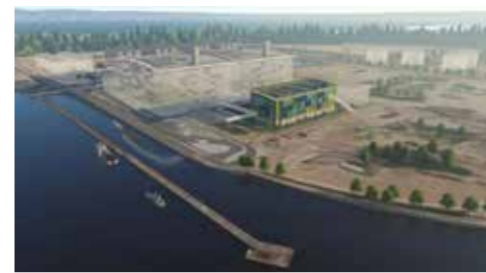
Photo CR: Masterplanning view - The National Environment Agency (NEA) and PUB, Singapore's National Water Agency
