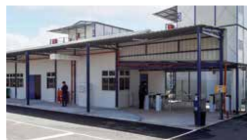
Tuas South Boulevard Dormitory
