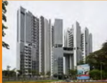
SILVERSEA, SINGAPORE Mechanical & Electrical Engineering
